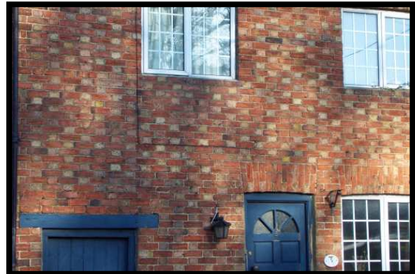
Photo 20 Basketwork brick bond of cottages on Greenside A4
