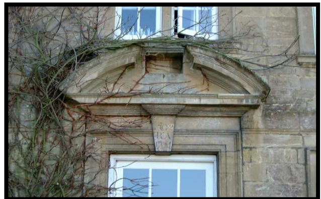
Photo 18 Wappenham House, detail of stonework
