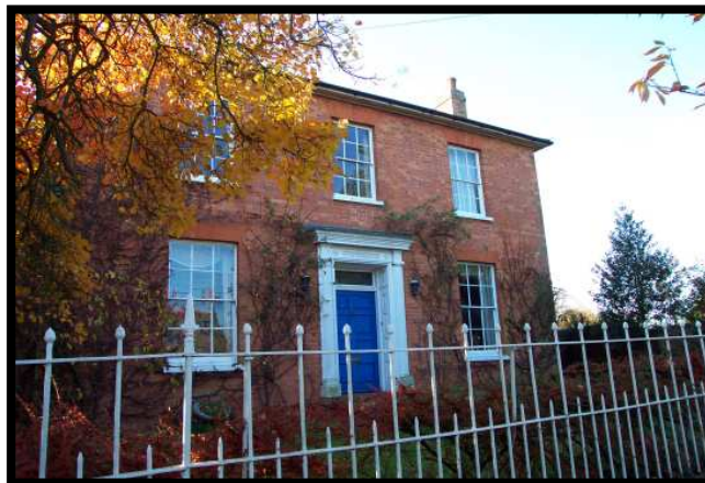
Photo 29 Iron railings at The Old Rectory may be original to the house
