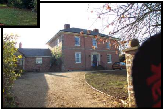
Hipped roof of High Street House →
